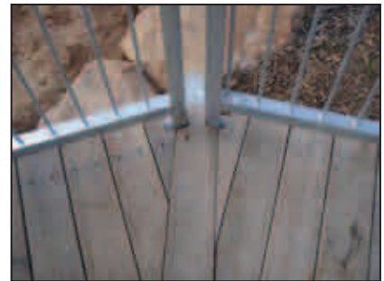
- Oran Park Town OSD4 deck
