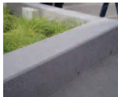
- Example of In situ wall character
