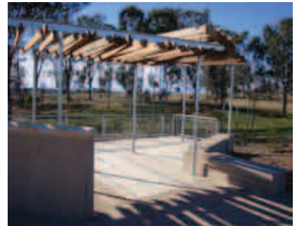
- Oran Park Town OSD4 deck
