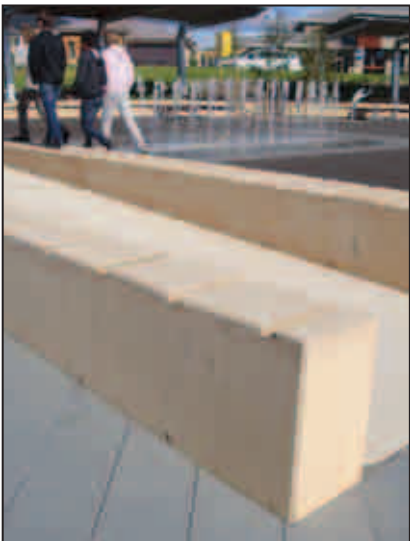
- Cast In-situ walls
