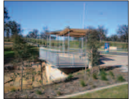
- Oran Park Town OSD4 deck
