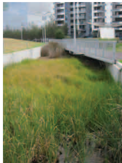
- Example of rain garden (Melbourne, Docklands)
